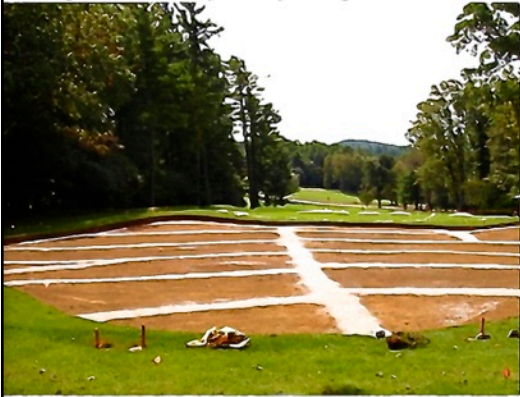
7. Fillpad ready to Float Out & Contour Green's Mix
