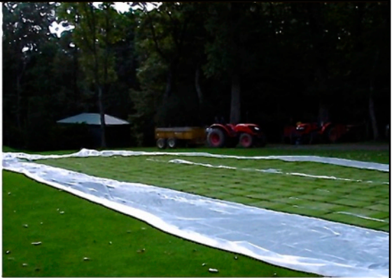
3. Stockpile Sod to the Side for Re-use
