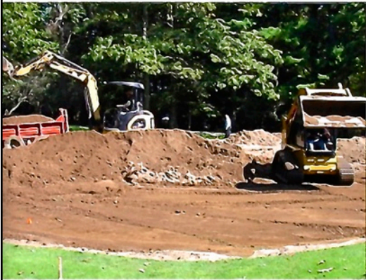
4. Scraping Away Decades of Topdressing and Organic Build-up Comprising the Inner Lift.
