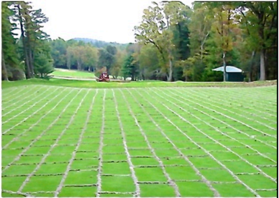
9. Filling the Seams with Rootzone Mix
