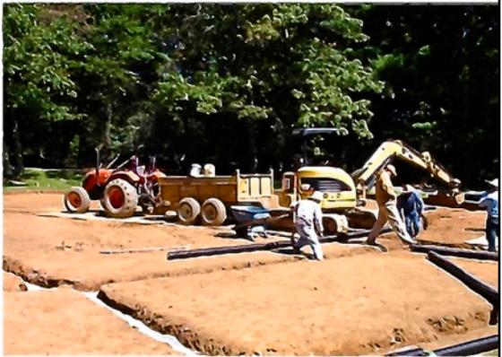
6. Installing Drainage in Sub-base Floor
