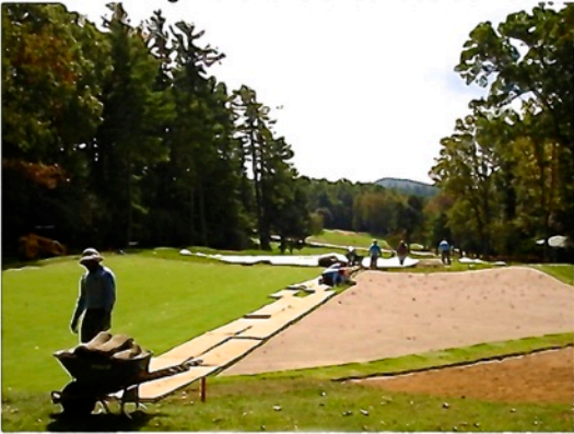
8. Replacing Old Sod & Supplementing Expansion with New
