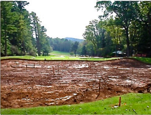
5. Coring Out Fillpad to Expanded Perimeters and Marking Elevations of Surface Contours
